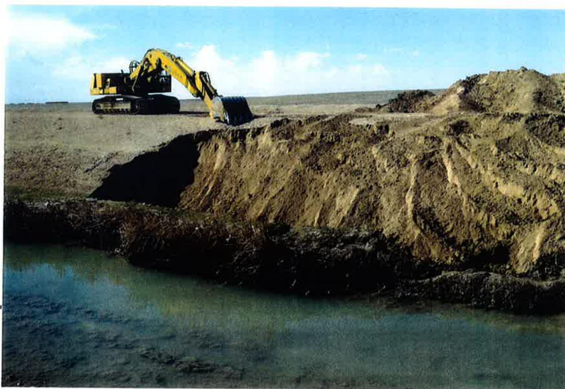
Feb 99: UNEX work on very wide silt shoulder near Marja siphon at Km 58+350. Remaining silt island was removed by hand labor.
