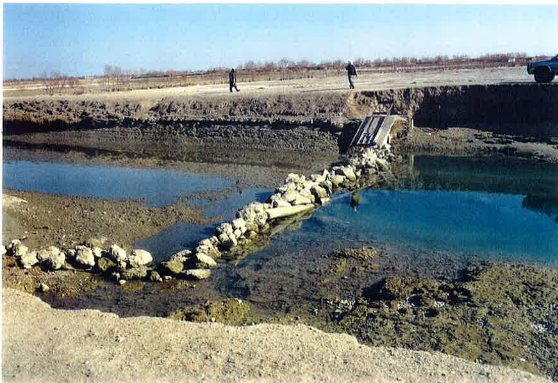
Feb 99: Before and After - Repairs at intake Km 47, Nad-i-Ali. Villager-built stone diversion wall was placed during water-short period of Boghra Canal.
