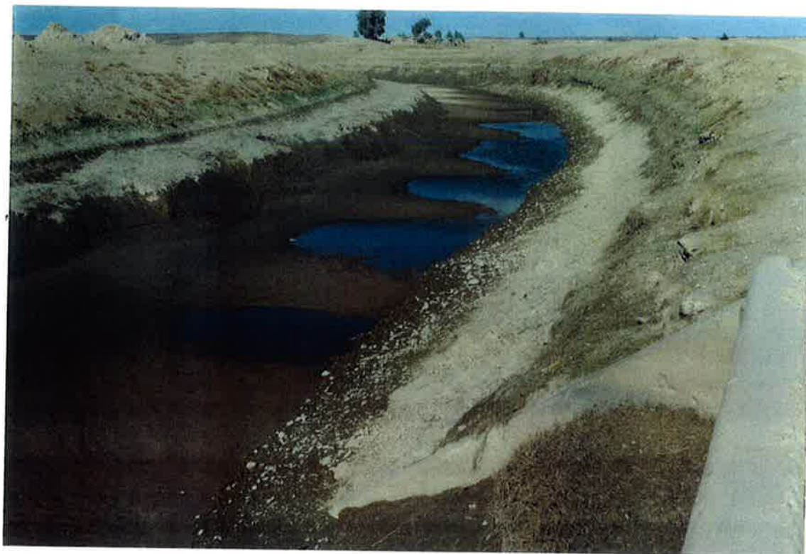
Feb 99: Marja Boghra Canal in drift area. Note sediment formations in the bottom of canal.
