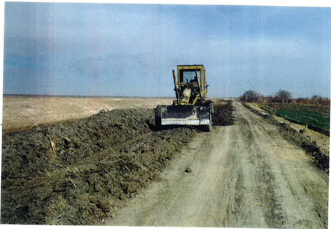
Feb 1999: MCI grader spreading the spoils of hand labor desilting on Nad-i-Ali service road.
