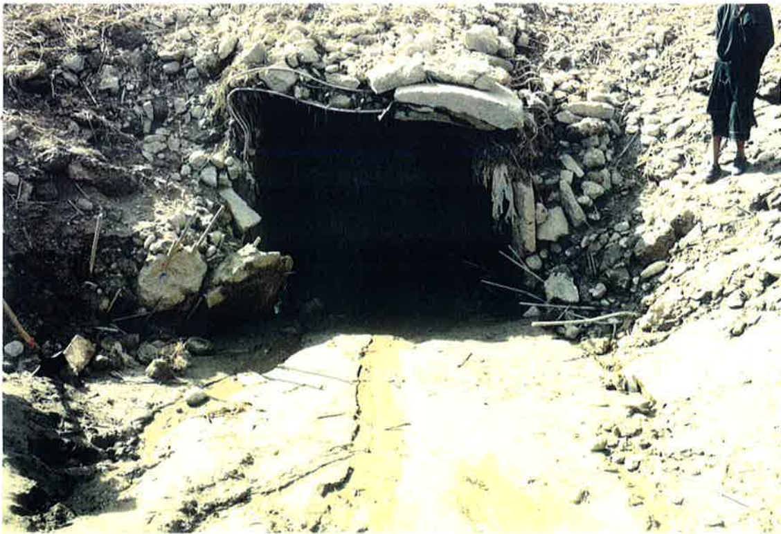
Damaged Marja siphon intake
