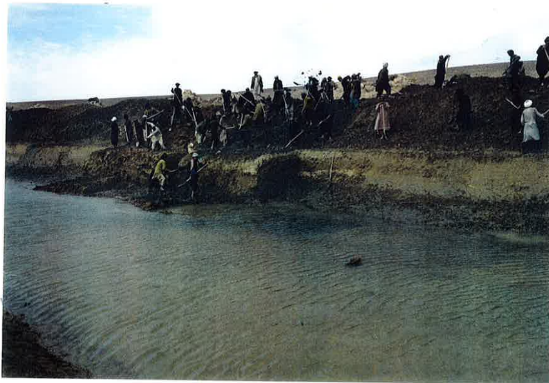
Feb 99: Silt being relayed; note cut of silt shoulder.
