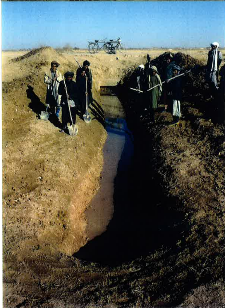
Jan 99: Before and After but not yet completed; Desilting underdrain Km 51+818 in Nad-i-Ali, desert side.
