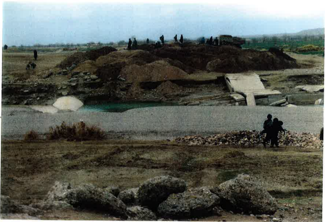
Feb 99: Damaged Ab Pashak exposed siphon under repair at Km 15+325
