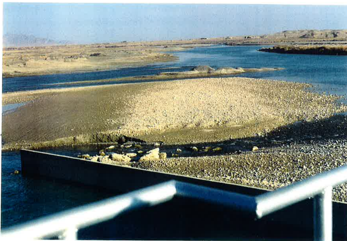
Jan 99: Boghra Canal intake area needing desilting; gravel delta in foreground.
