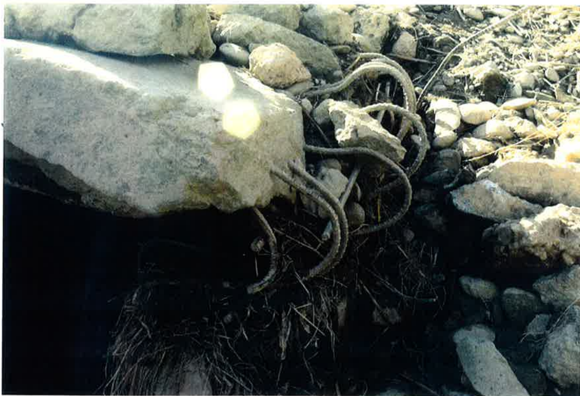
Detail of damaged Marja siphon intake top right corner
