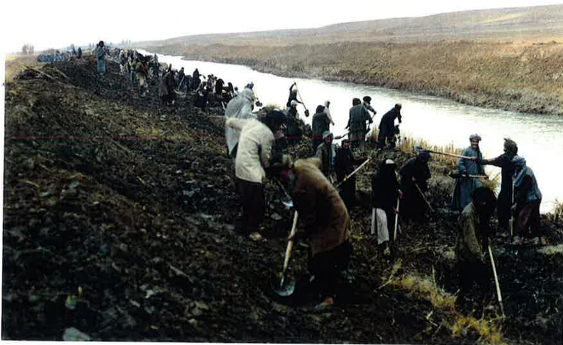
Feb 1999: Work on wide silt shoulder in Nad-i-Ali at Km. 50
