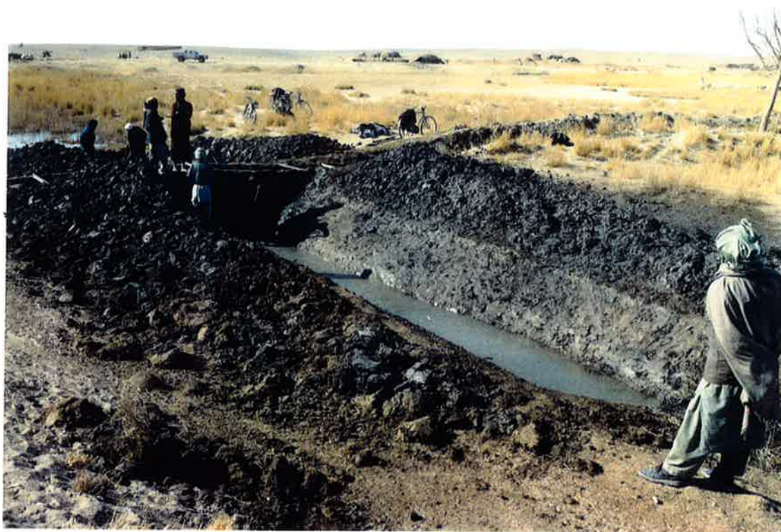
Jan 99: Before and After views - desilting drain under farm ditch near underdrain at Km 51; Nad-i-Ali
