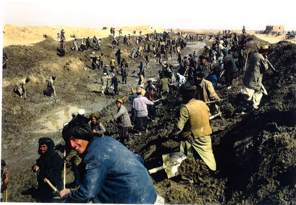
Feb 99: Desilting of Boghra Canal sides and bottom near siphon at Km 73+962
