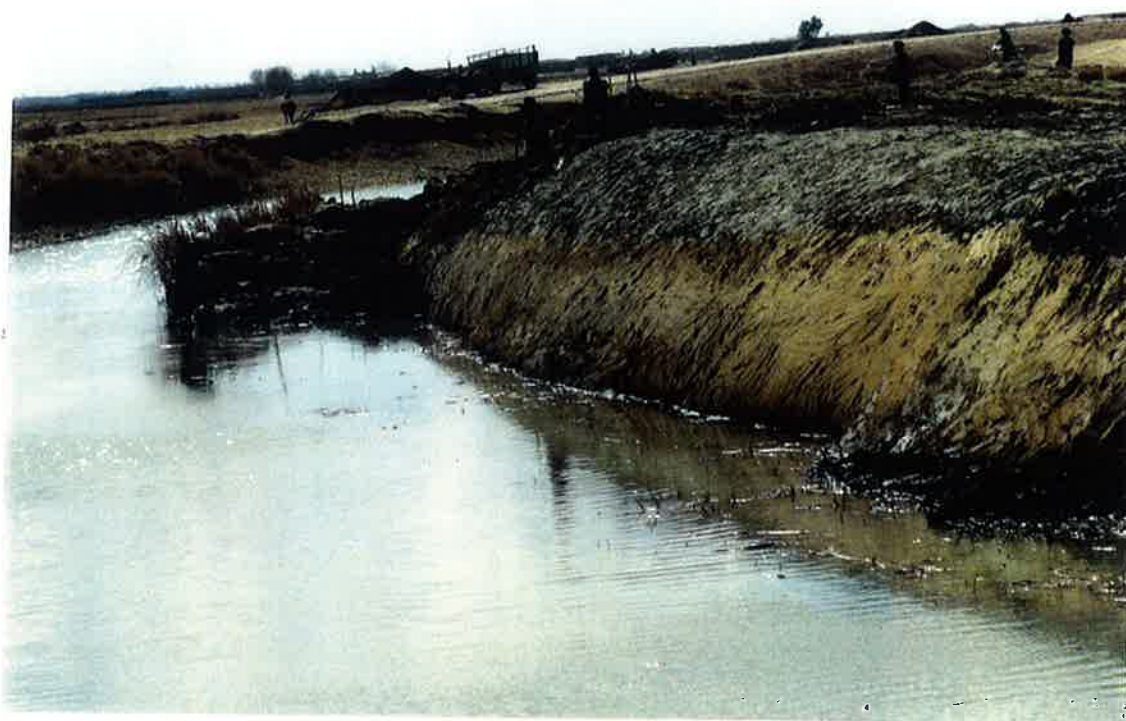
Feb 1999: Completed segment of embankment. Note remaining shoulder of silt awaiting canal re-closure; Nad-i-Ali at Km 55+300.
