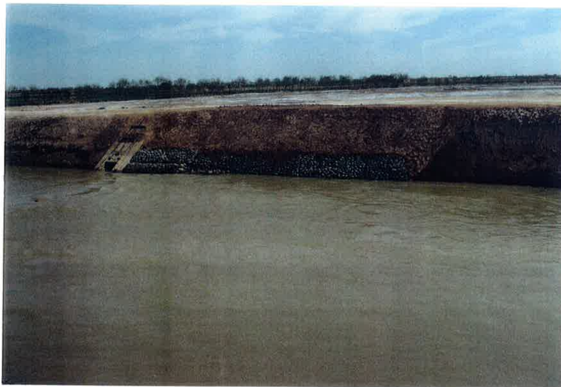
Feb 99: Before and After - Repairs at intake Km 47, Nad-i-Ali. Villager-built stone diversion wall was placed during water-short period of Boghra Canal.
