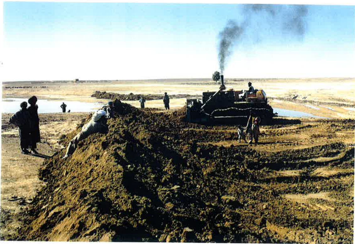
Feb 99: Before and During - repair of 695 meters of old MKA diversion dikes at siphon 46+767
