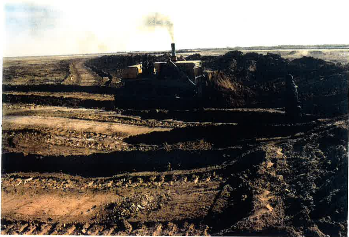
Feb 99: Before and During - repair of 695 meters of old MKA diversion dikes at siphon 46+767
