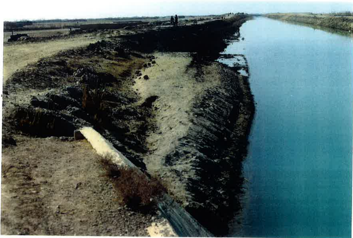
Jan 99: Before and After -- desilting of silt shoulder at Loy Manda siphon exit at Km 29+865
