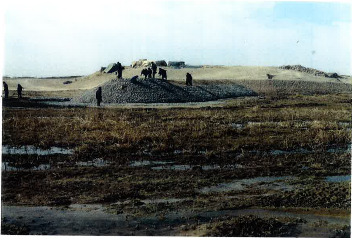
Feb 99: Gabion-protected Loy Manda siphon barrel nearing completion.
