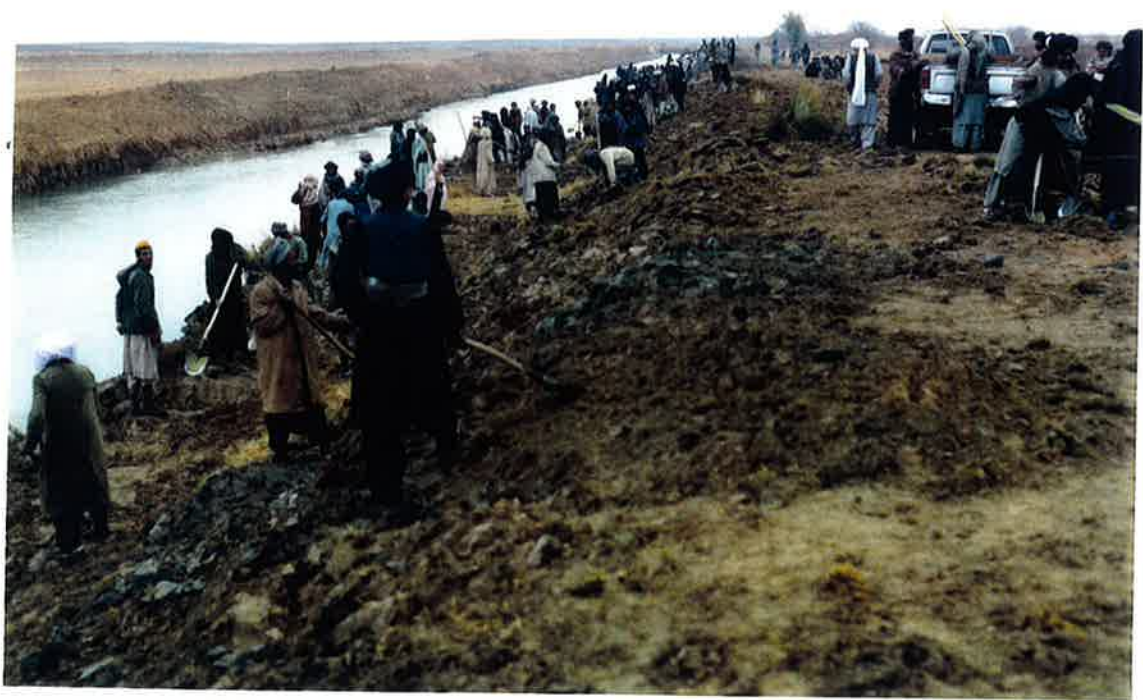
Feb 1999: Boghra Canal hand labor force, Nad-i-Ali; Men working on silt shoulder 6-8 feet wide.
