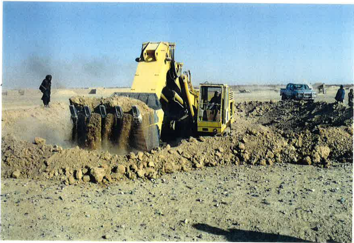
Jan 99: HAVA heavy equipment excavating fill for Loy Manda siphon
