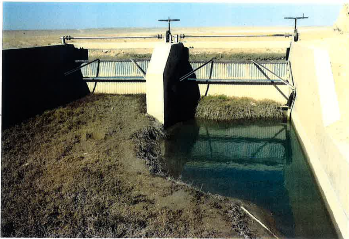
Feb 99: Silted wasteway and gates at Km 46+617; work interrupted by land mine discovery.
