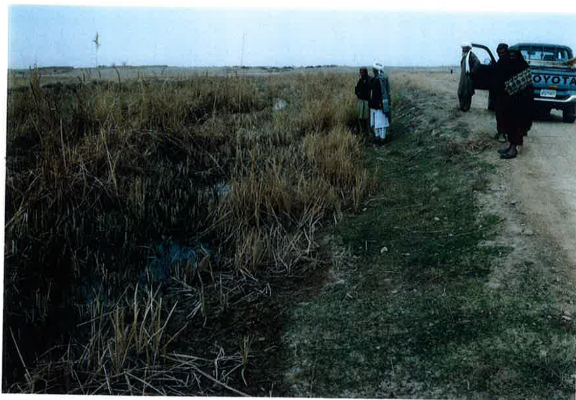
Mar 99: Silted wasteway with growth at Km 70+60, Marja
