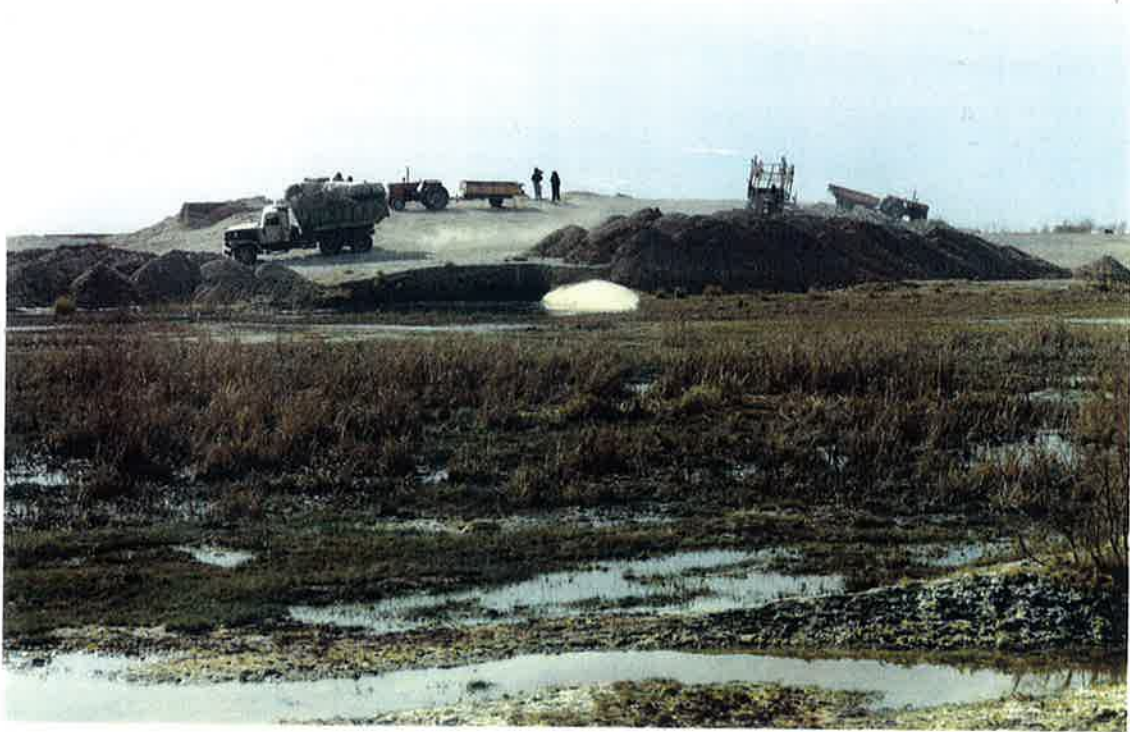
Jan 99: Loy Manda siphon under repair; exposed siphon barrel in center.
