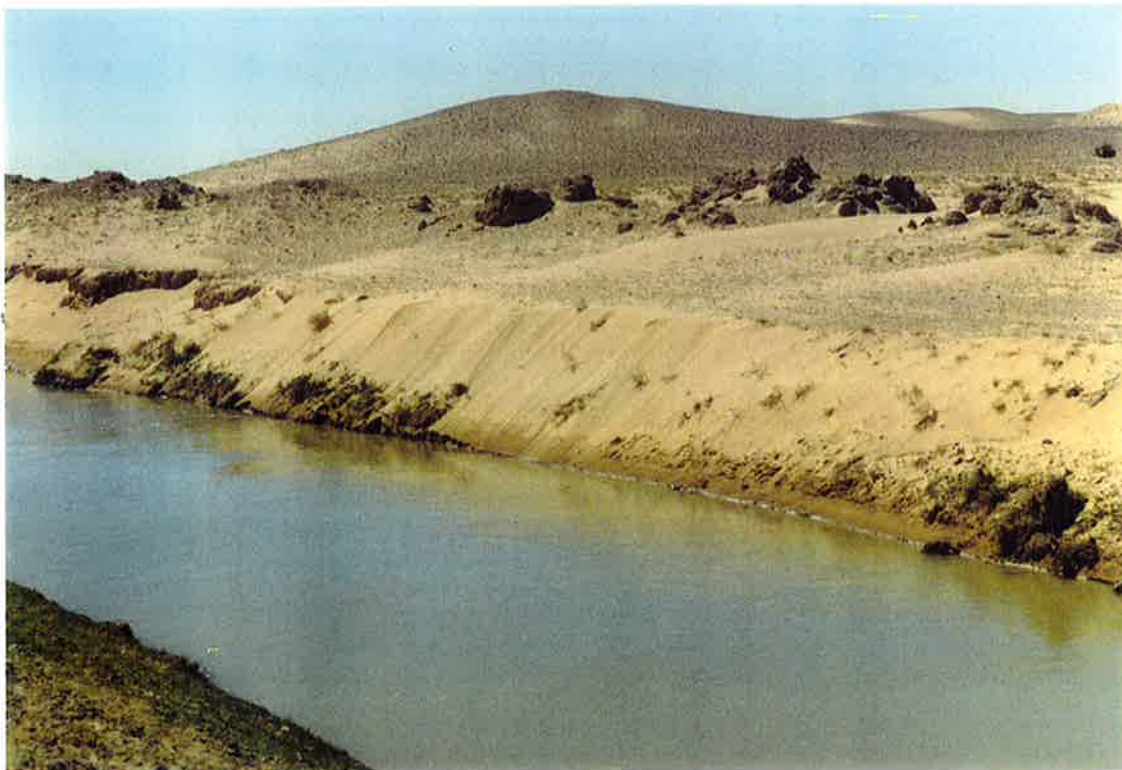
20 Mar 99: East Marja Branch of Boghra Canal with blown sand from desert.
