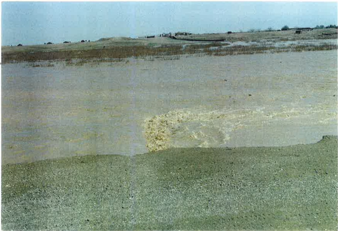
18 Mar 97: Rough water excavating Loy Manda siphon barrel at Km 29+865
