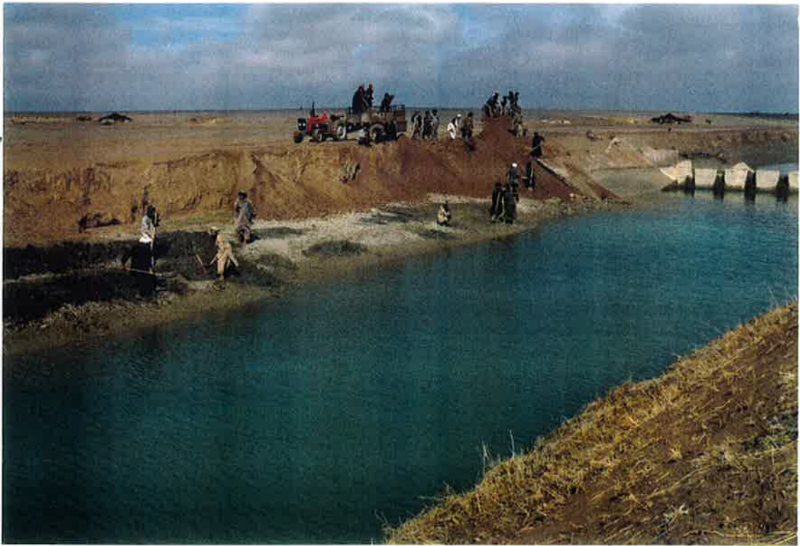
Feb 99: Before and After - repairs at drop structure Km 47+650, Nad-i-Ali
