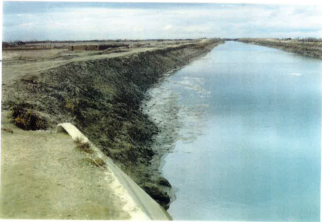
Jan 99: Before and After -- desilting of silt shoulder at Loy Manda siphon exit at Km 29+865
