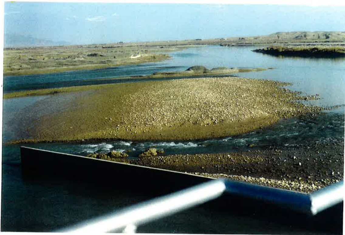
Jan 99: Gravel delta at Boghra Canal intake
