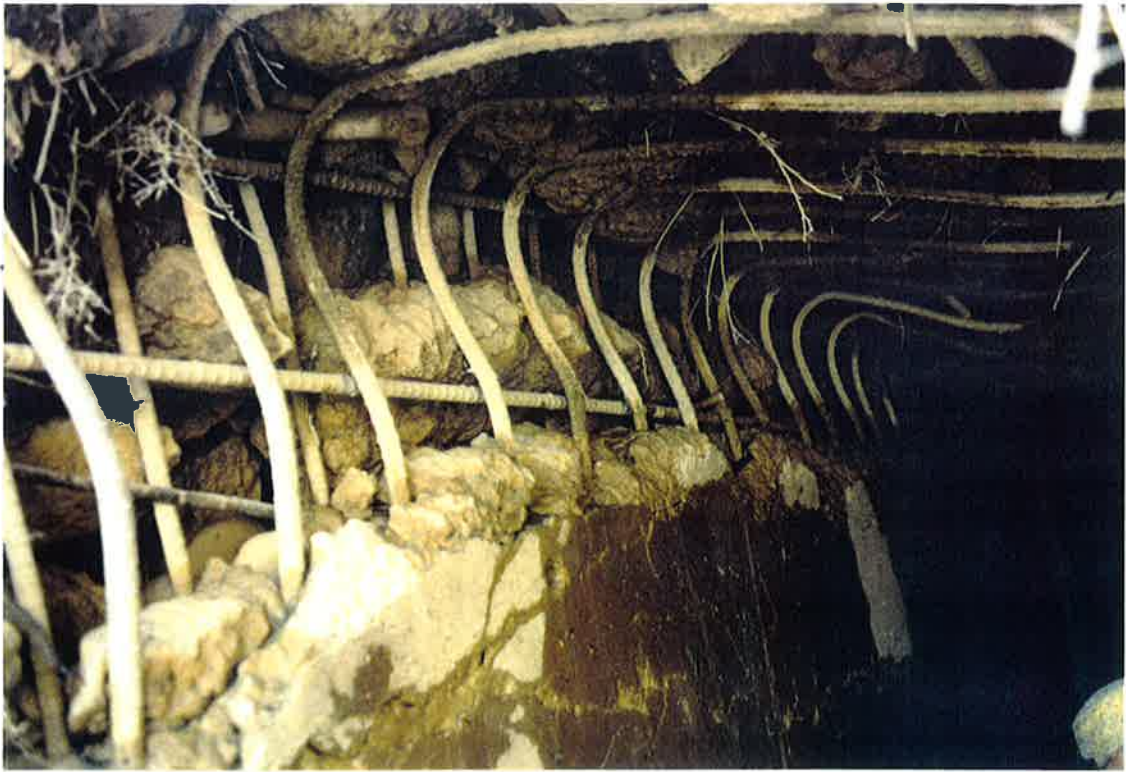
Detail of damaged Marja siphon intake top left corner, inside
