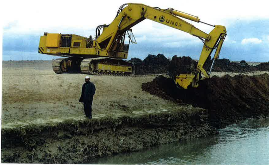
Feb 99: UNEX work on wide silt shoulder near Marja siphon at Km 58+350.
