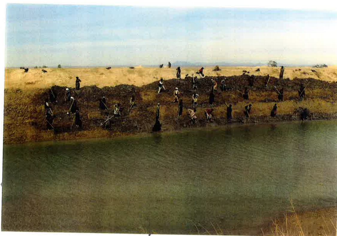
Feb 99: Silt being relayed up and out of the Boghra Canal in Marja; near Km 68.
