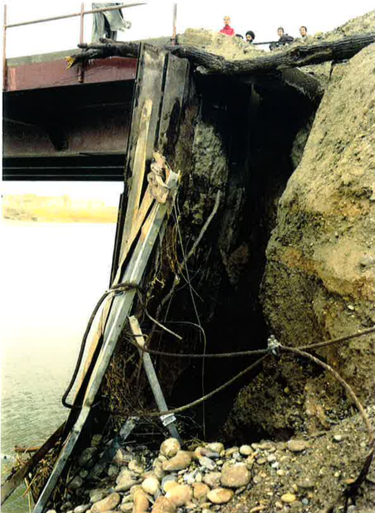
Damage at Lashkar Gah Bridge from flood of 7 Feb 99
