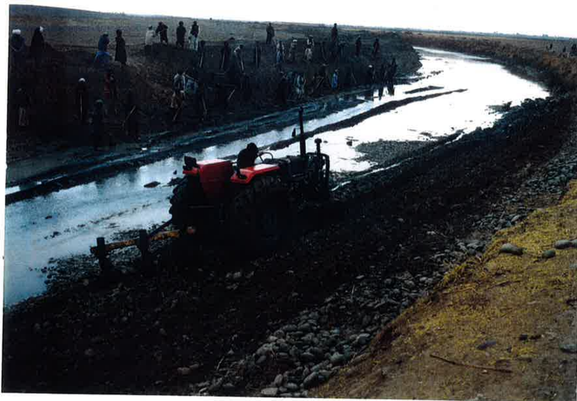
Feb 1999: Local tractor with plow loosening compacted clay silt; Nad-i-Ali at Km. 55+400.
