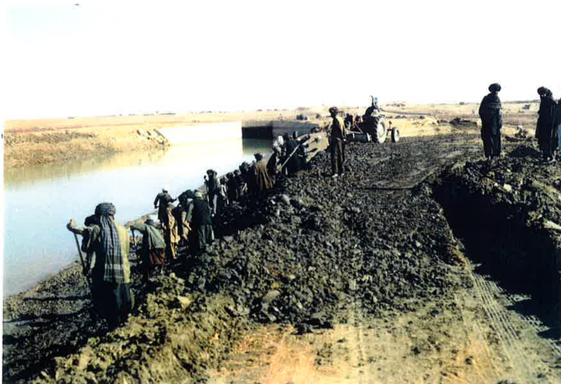
Jan 1999: Tractor spreading the spoils of hand labor desilting near Loy Manda siphon at Km: 30+355.
