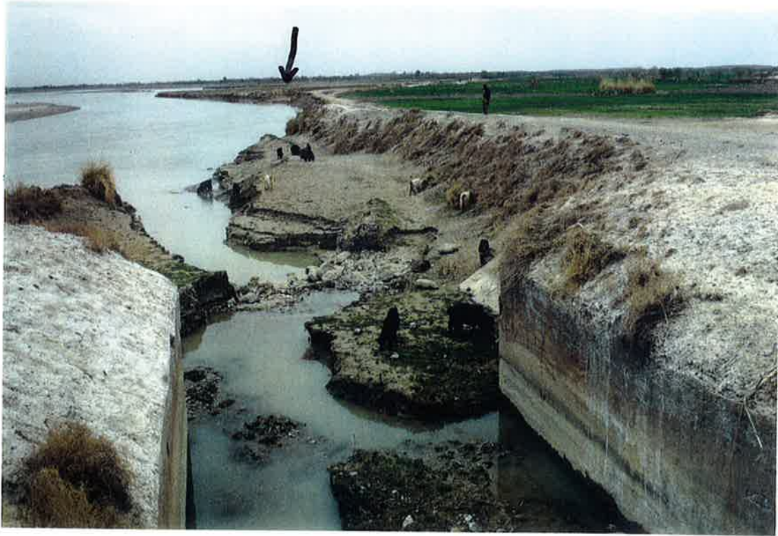
Jan 99: Shamalan Canal washout #2 Above photo from wasteway #1 looking south; Below photo from canal looking north at wasteway #1
