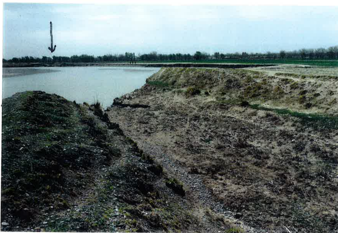
Jan 99: Shamalan Canal washout from the north; arrow indicates other end of washout.
