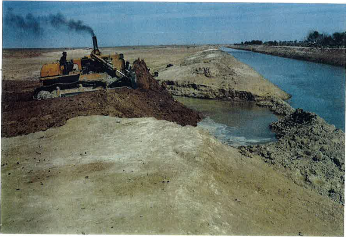
Feb 99: Before and After - repair of broken canal embankment; Km 48, Nad-i-Ali
